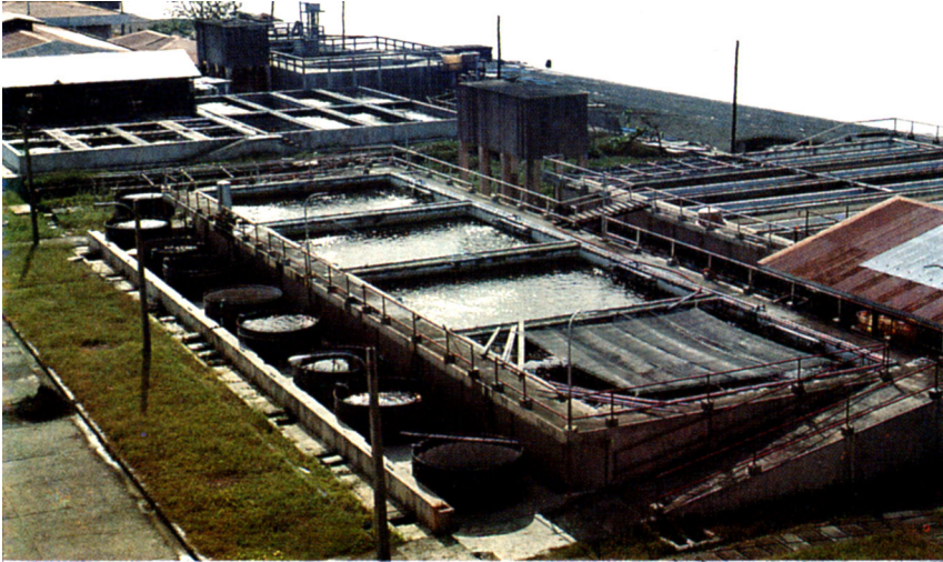
Fig. 7. Concrete tanks for milkfish broodstock at SEAFDEC/AQD's Tigbauan Main Station.
